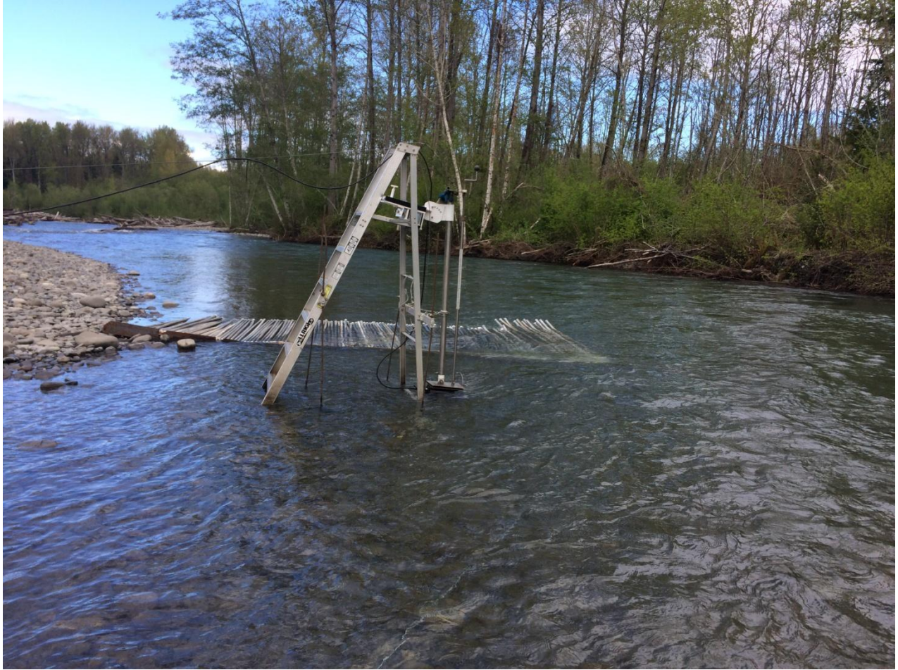
Figure 2. Photo of the HRC DIDSON site showing the picket weir and the ladder on which the DIDSON is mounted.
